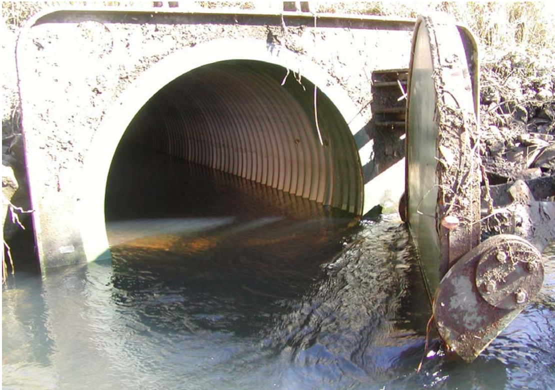
Figure 7. Open Tide Gate at W201+30 Slough
